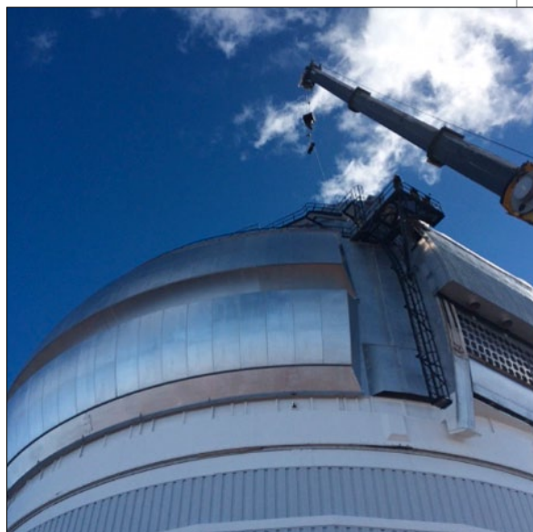
Figure 2. Hoisting a 150-pound drive motor, using one of the largest cranes available on the island of Hawai'i.
