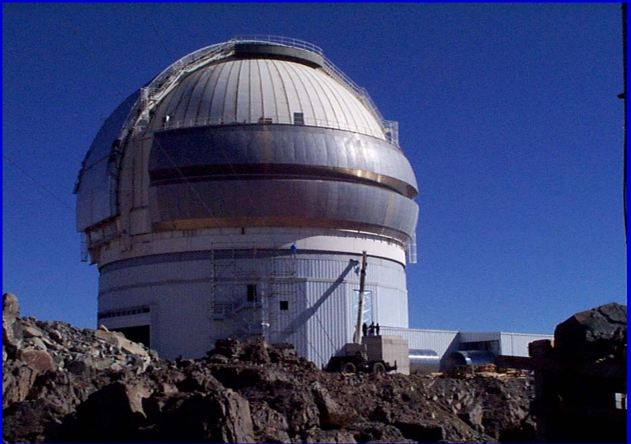
The completed Cerro Pachon enclosure, September 1998.
